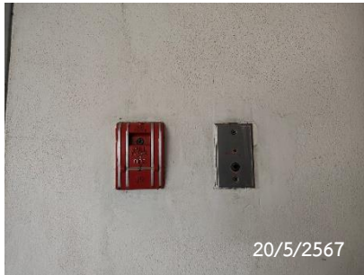
Fire Alarm Manual Station
